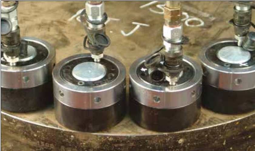
▲ Tensioning with hydraulic nuts.
